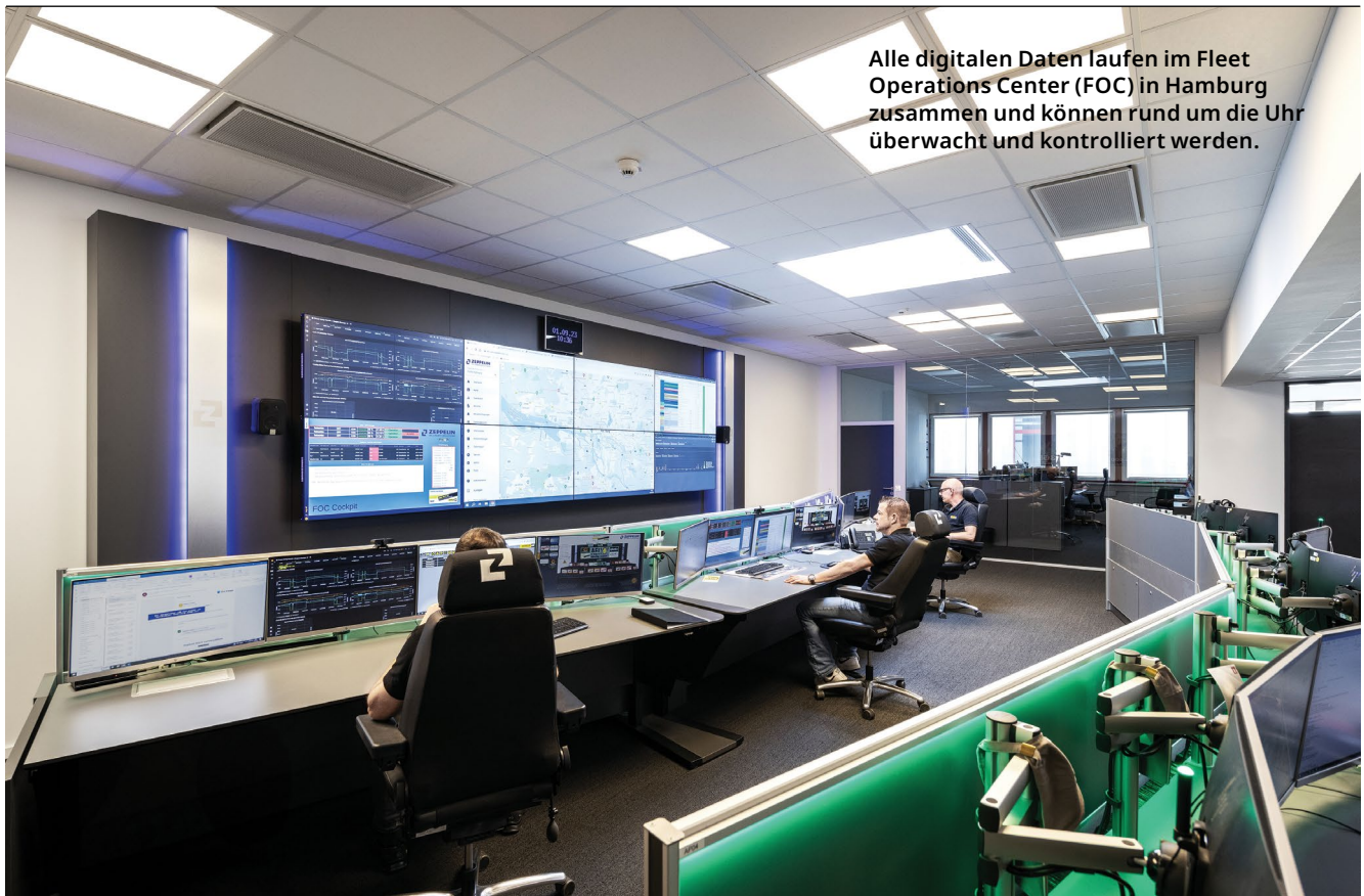
Zeppelin Power Systems
